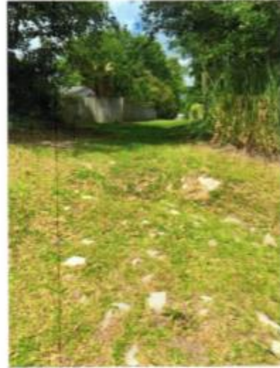
refresh rip rap at inlets and swales
